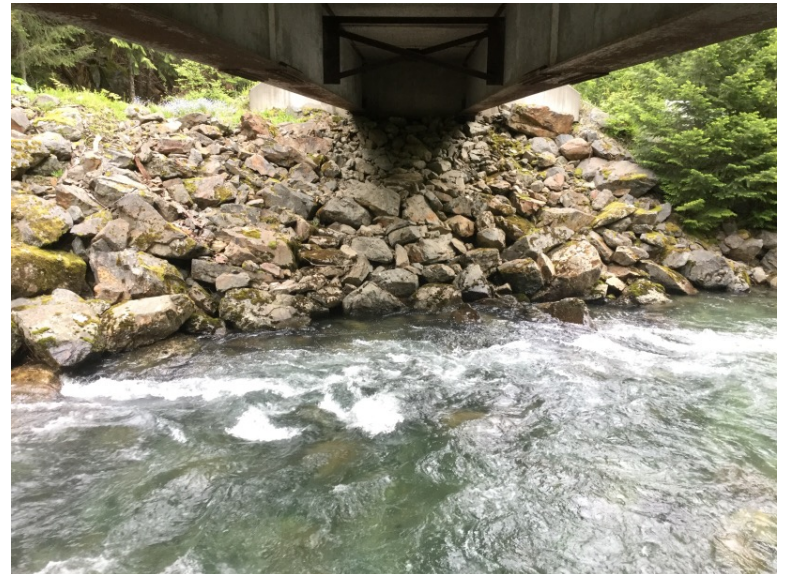
Left Bank Abutment when facing downstream
