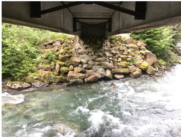
Right Bank Abutment when facing downstream
